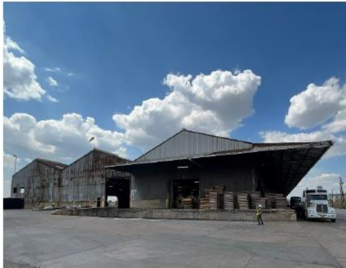
3 Overall view of the South Elevation (end of Shed 19).
