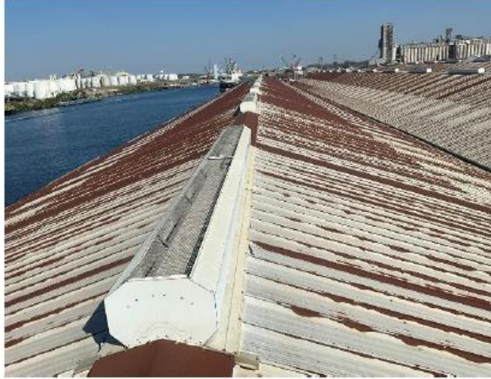
1 Overall view of Shed 18-19 roof (viewed towards Northwest).
