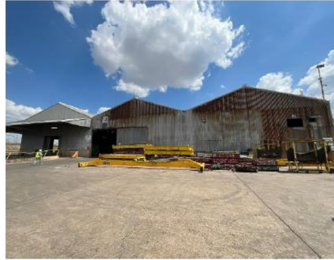
2 Overall view of the North Elevation (end of Shed 18).
