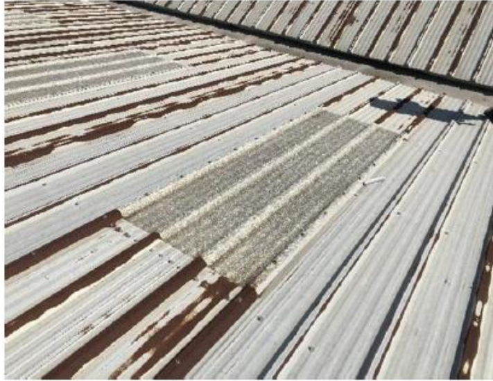
7 View of typical fiberglass lite panels.
