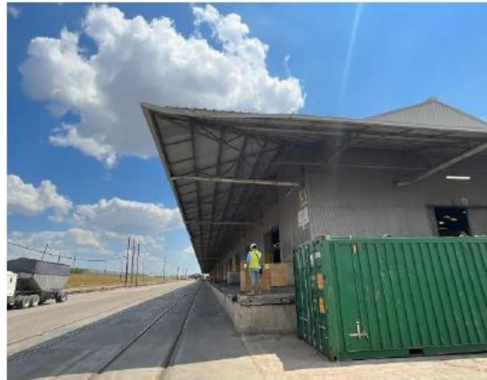
4 Overall view of the East Elevation (Land Side).
