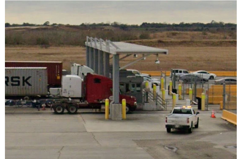
Existing TWIC Canopy
