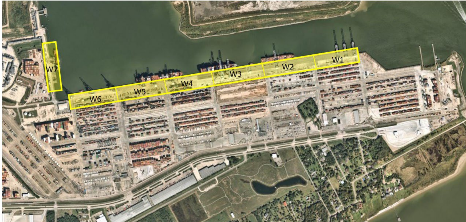
BARBOURS CUT CONTAINER TERMINAL
