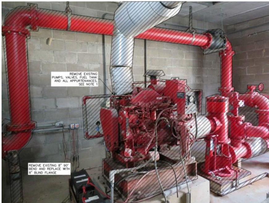
SALTWATER PUMP BUILDING DEMOLITION N.T.S.
