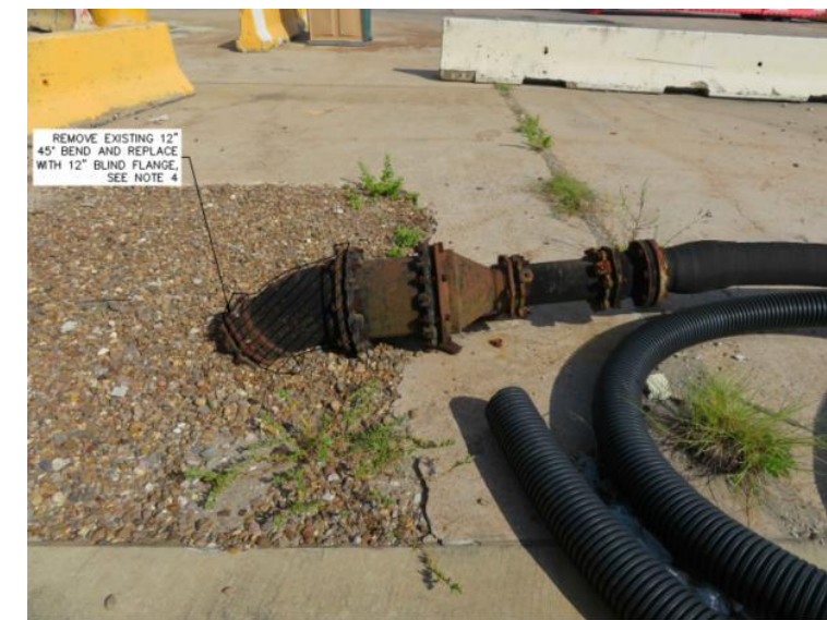
MOBILE SALTWATER PUMP CONNECTION N.T.S.
