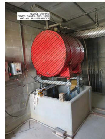
SALTWATER PUMP BUILDING DEMOLITION N.T.S.
