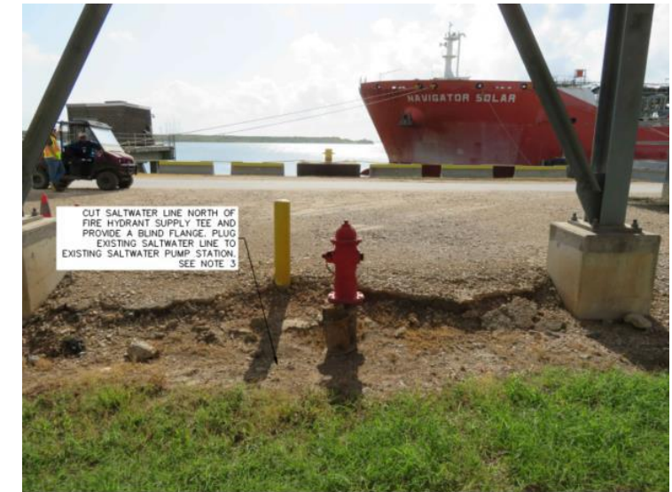
NORTH FIRE HYDRANT MODIFICATION N.T.S.
