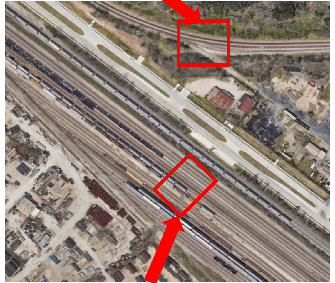
30" Steel Casing Repair
